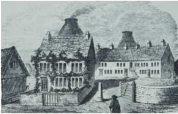
Abb.57: Ivy House Works
